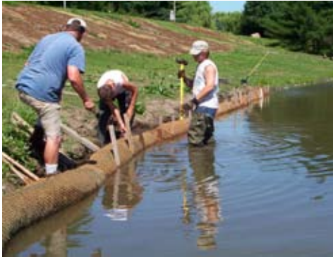
Installation of biologic materials for shoreline stabilization.
