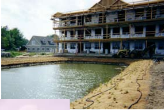
Shoreline stabilization for condominiums. (upper photo is during construction. Photo to the left is after vegetation is established.)
